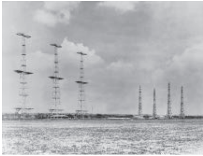
▲ Fig. 2 The Chain Home was the first British radar system, used during World War II to warn of approaching German aircraft. Source: Wikimedia Commons.
